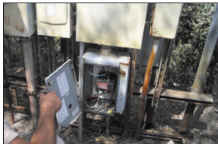
Photo 6: At this large strip shopping plaza the electrical control supports, panels, and conduits have rusted through. One panel door was rusted shut and fell off when our electrician finally managed to pry it open.
