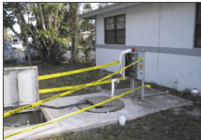
Photo 8: Another “temporary” bypass in a residential area in front of one-story condos. The valve pit, wet well, and control panel were all left open. City personnel added the caution tape when called out to the property by residents who stated that it had been in this condition for several weeks.
