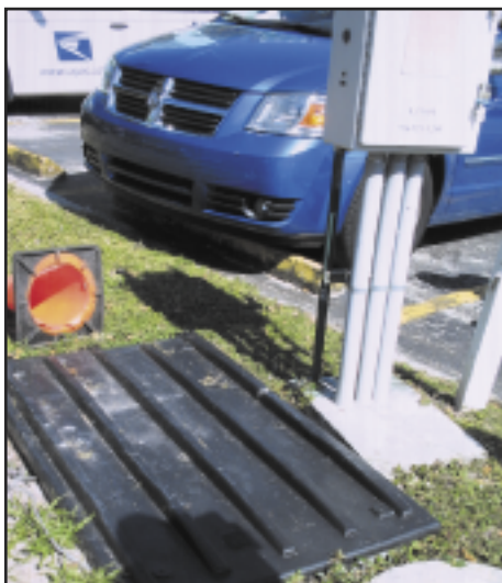
Photo 2: The flexible black plastic shown here is acting as a “temporary” wet well cover after the previous cover rusted through and fell into the wet well. The lift station is located in the front parking lot of a large condominium in a 55-plus community, presenting a substantial hazard to the seniors who live there. “Temporary” in this case was several months, according to residents.
