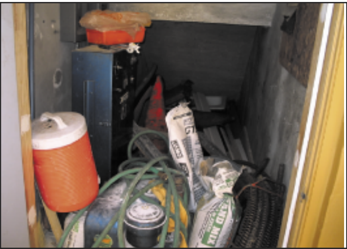
Photo 11: Here a control panel is located inside a storage room to protect it from the elements. The panels are inaccessible because of the large quantity of stored items in the closet. This also illustrates how infrequently these systems are tested or checked for damage.
