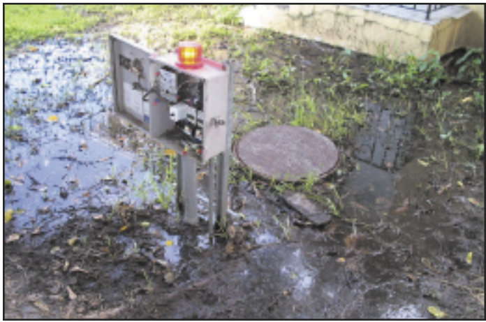
Photo 10: Flooding around an overflowing lift station. The light was on and the panel was open as shown when city personnel arrived, but no maintenance crews were onsite. Home and condo owner associations frequently rely on their regular maintenance staff, who have little or no training, for the upkeep of their private lift station. Staff members may not even be aware of the equipment's purpose.
