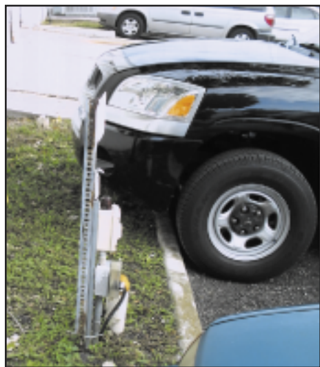
Photo 1: This photo of a private lift station electrical control panel located adjacent to a parking lot shows several cars pulled up even with the panel. If either vehicle had parked farther to the side, substantial damage to the lift station, as well as an electrical hazard, would have resulted. This illustrates the importance of protecting private lift station systems from vehicular traffic.
