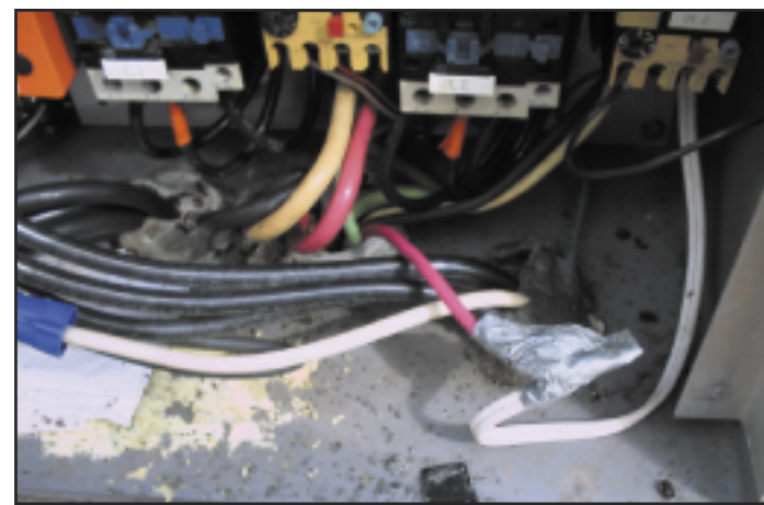
Photo 7: Inside another electrical control panel, wires have been spliced and covered with duct tape. Copious quantities of rodent feces inside the box may indicate the reason for splicing.
