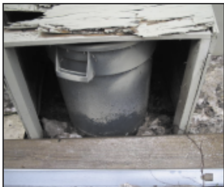
Photo 3: At this shopping center parking lot, several planks and pieces of shelving were used to cover a pit dug by maintenance crews while repairing damaged sewage lines to a private lift station.
