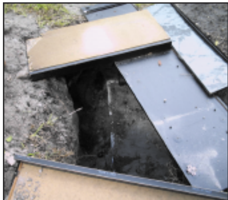
Photo 3: At this shopping center parking lot, several planks and pieces of shelving were used to cover a pit dug by maintenance crews while repairing damaged sewage lines to a private lift station.
